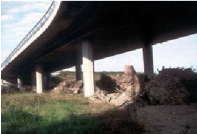
Figure 6.23: Underpass to accommodate large and medium mammals, with stumps and vegetative cover for small animals (FHWA/US DOT, 2002)
