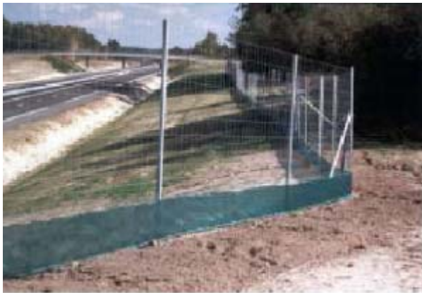
Figure 6.2: Wide mesh chain fence for large mammals, with a fine mesh fence border for small mammals and amphibians (FHWA/US DOT, 2002)
