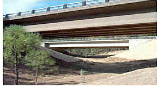
Figure 4.2: Underpass with open field of view for large mammals
