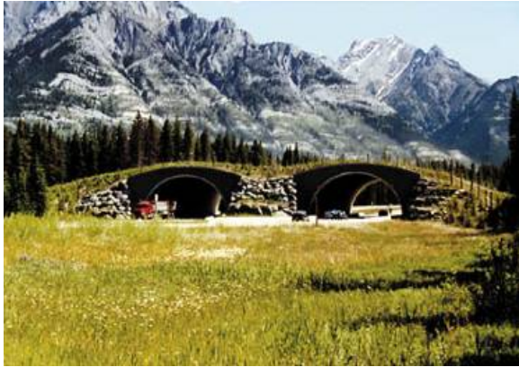
Figure 6.28: Overpass in Banff National Park, Canada (CPAWS, 2004)
