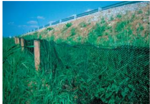
Figure 6.3: Fine plastic mesh fence for small animals and amphibians (Puky, 2003)
