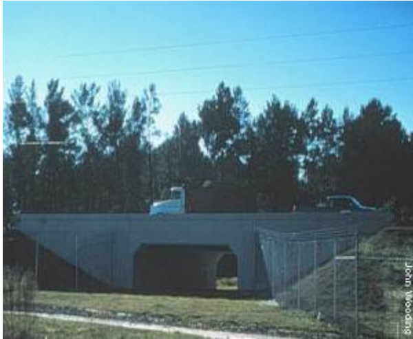
Figure 6.15: Fenced underpass for large wildlife (Defenders of Wildlife)
