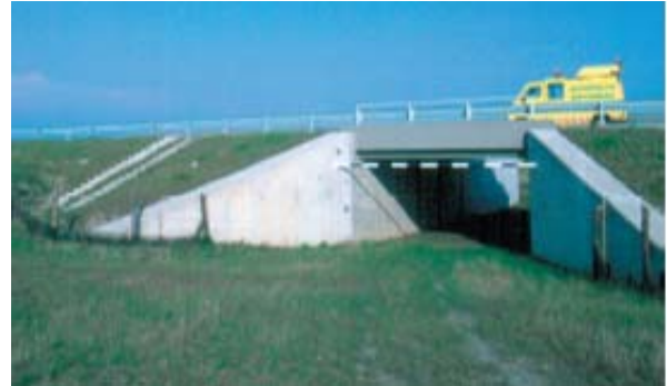
Figure 3.8: Box Culvert
