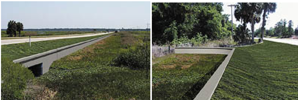
Figure 6.7: Lipped walls for amphibians (Critter Crossings Website, 2002)
