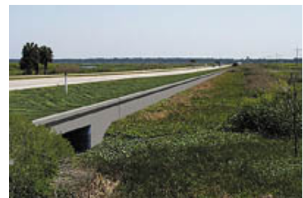
Figure 3.2: Lipped concrete wall
