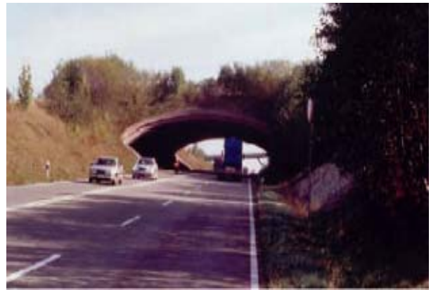
Figure 6.29: Wildlife overpass (Deer-Vehicle Crash Information & Research Center)
