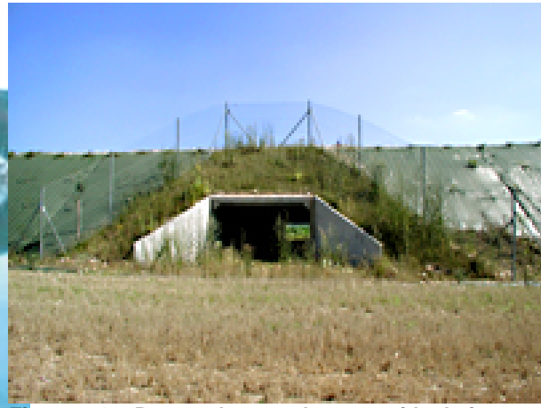
Figure 6.18: Box culvert underpass with chain link fence for large animals (Cemagref, 2002)
