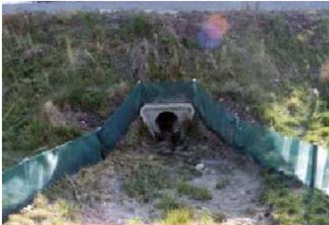
Figure 6.9: Small pipe culvert with mesh fence for small mammals and amphibians (FHWA/US DOT, 2002)
