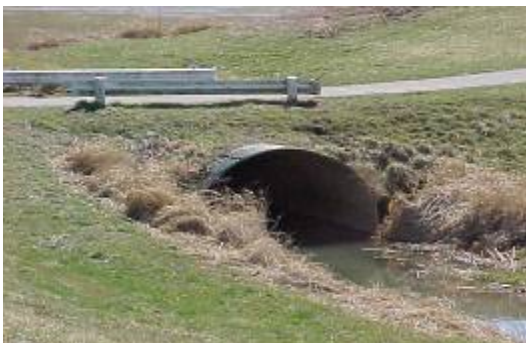
Figure 3.5: Culvert with standing water.
