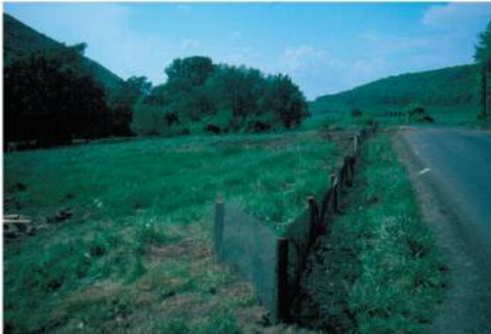
Figure 6.6: Fence for small animals and amphibians with turned-back end to prevent animals from approaching the road (Puky, 2003)
