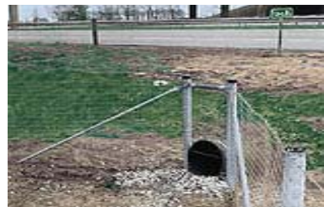
Figure 3.7: Pipe culvert
