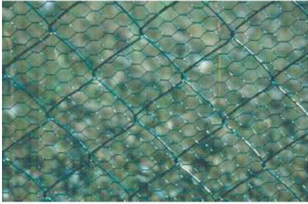
Figure 6.4: Chain link fence for large animals overlaid with fine plastic mesh fencing for small animals and amphibians (Puky, 2003)
