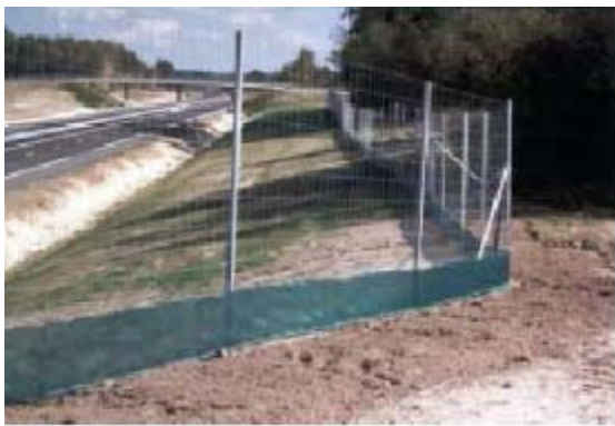
Figure 4.5: Wide mesh chain fence for large mammals, with a fine mesh fence border for small mammals and amphibians (FHWA/US DOT 2002)
