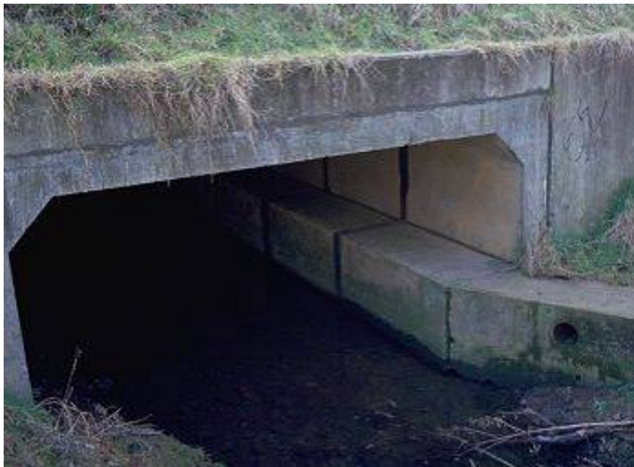
Figure 6.22: Box culvert modified with ledge for small animal passage (Jackson, 2004)
