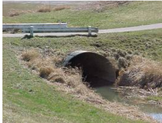
Figure 6.42: Culvert with standing water.
