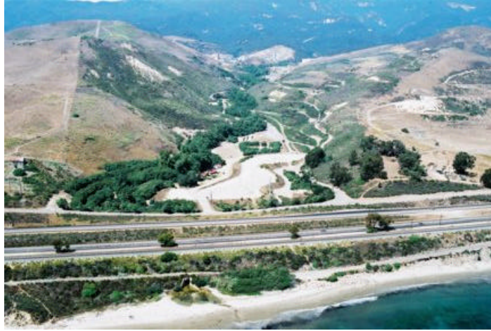
Figure 7.8a Highway 101 and UPRR culvert crossing at Corral Creek
