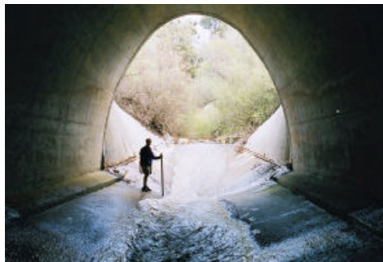
Figure 1.3.1 Rincon Creek Highway 101 Culvert
