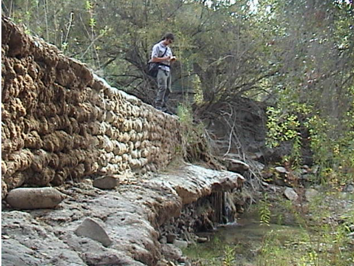
Severe undercutting
