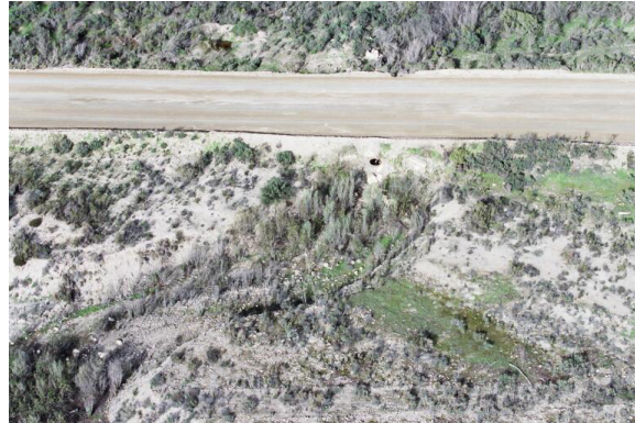
View Looking North (upstream) at SC_TT_1 culvert
