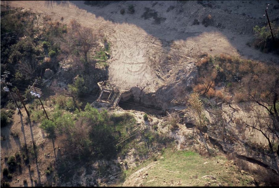
Old structure (SC_PU_LE_3) on Lime Creek
