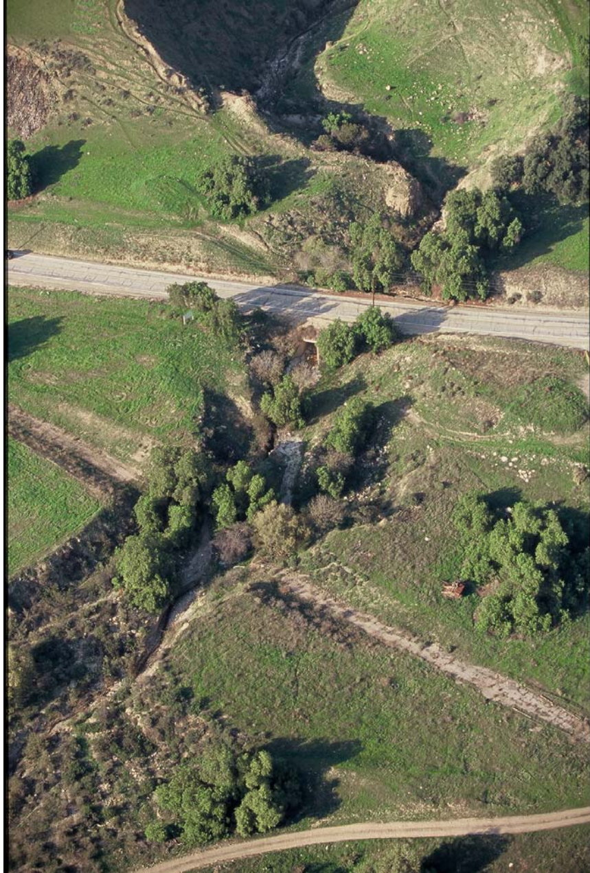
Piru Canyon Road Box Culvert SC_PU_MO_1 on Modelo Creek
