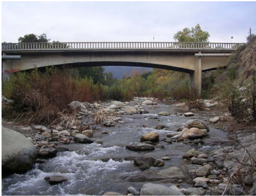
Santa Paula Creek at Steckel Park Bridge
