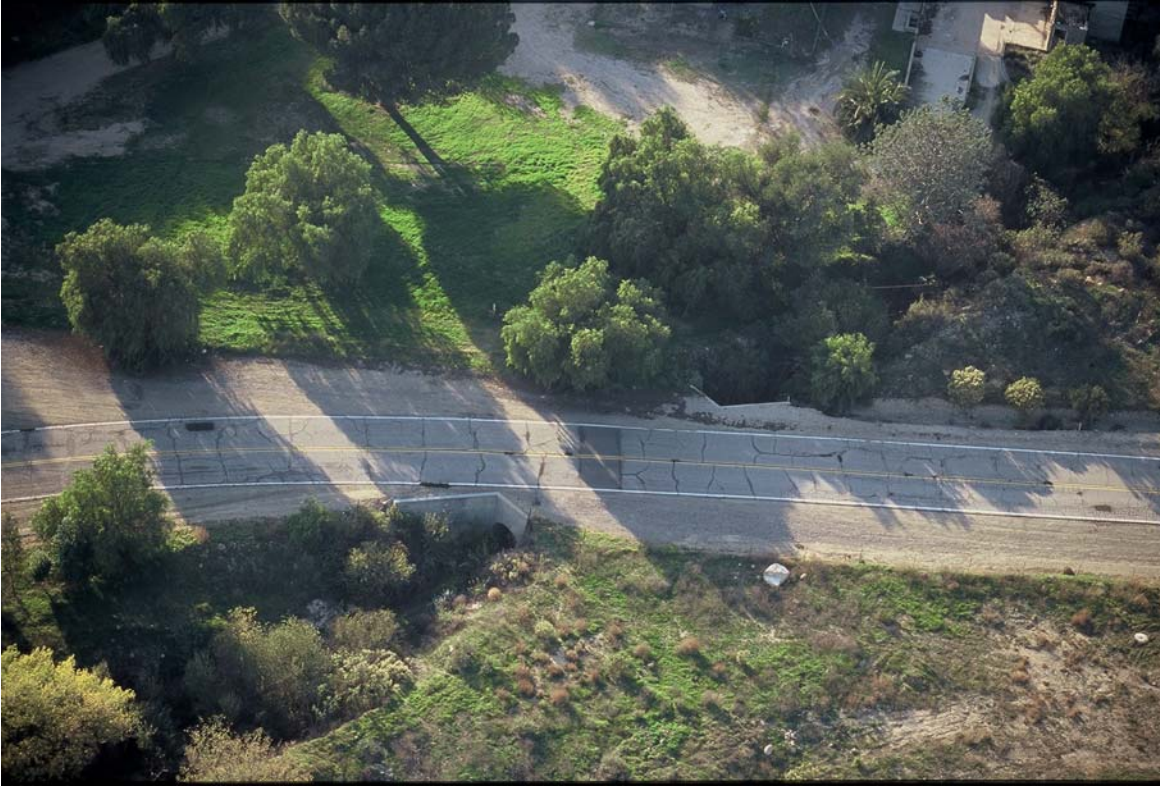
Piru Canyon Road Culvert (SC_PU_LE_2) on Lime Creek
