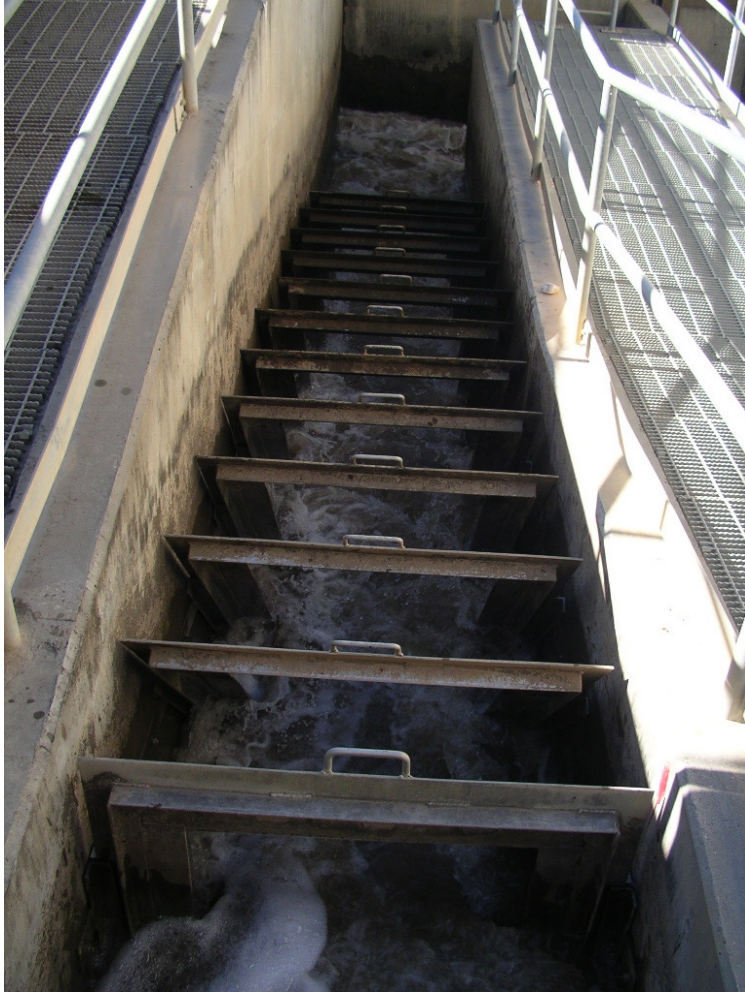
Denil Fishway at the Vern Freeman Diversion
