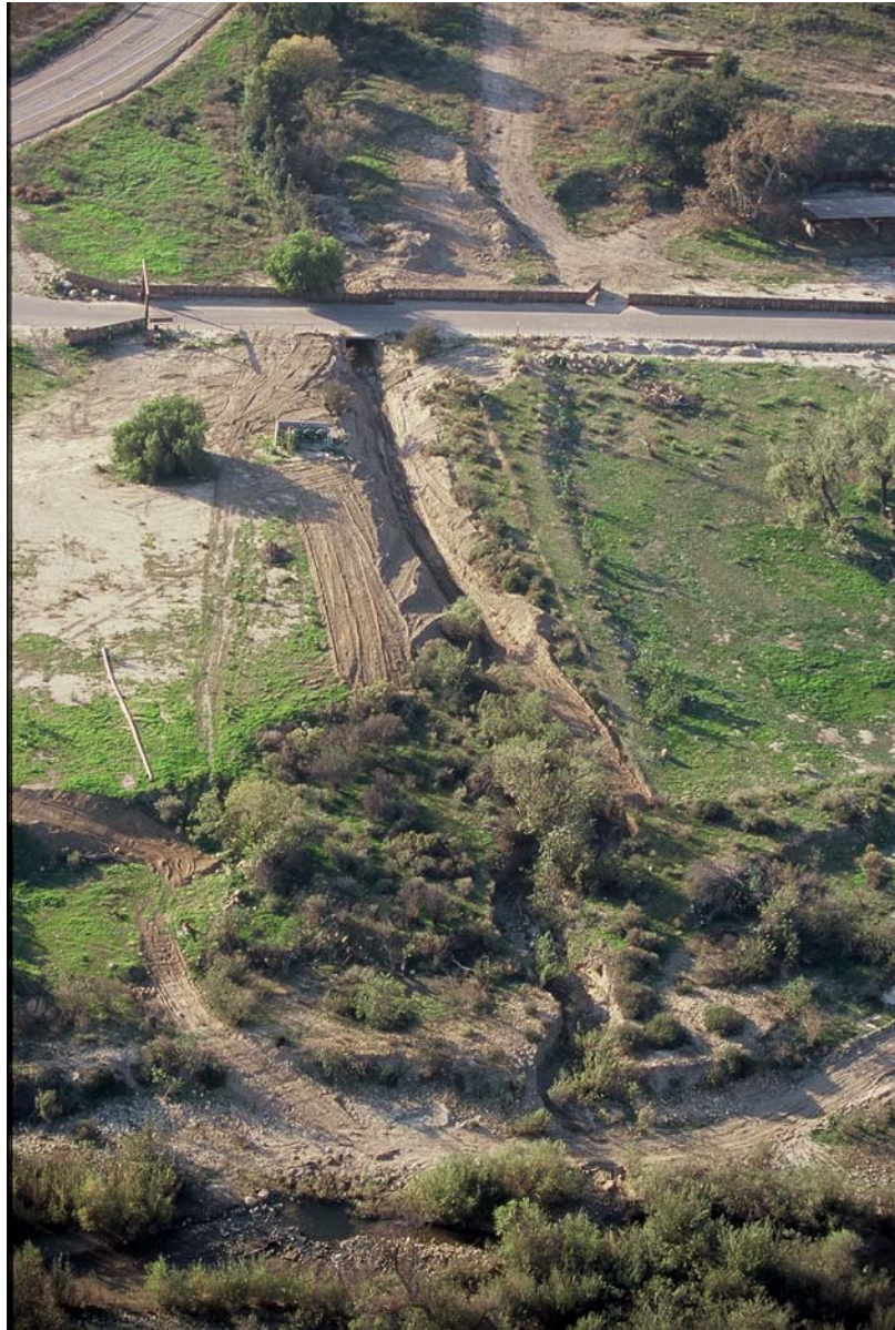
Private Box Culvert (SC_PU_LE_1) on Lime Creek
