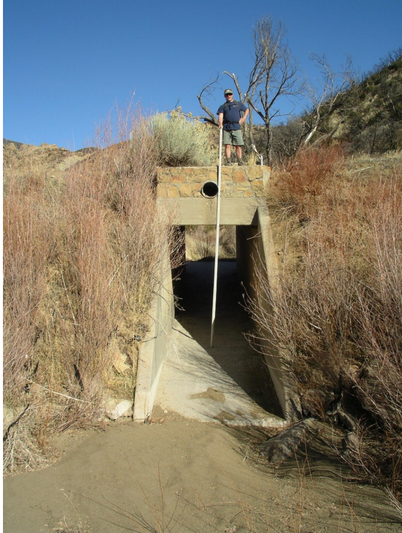
Burro Creek #2 Highway 33 Box Culvert
