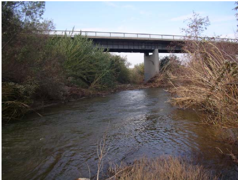
Downstream of the Santa Paula Creek confluence
