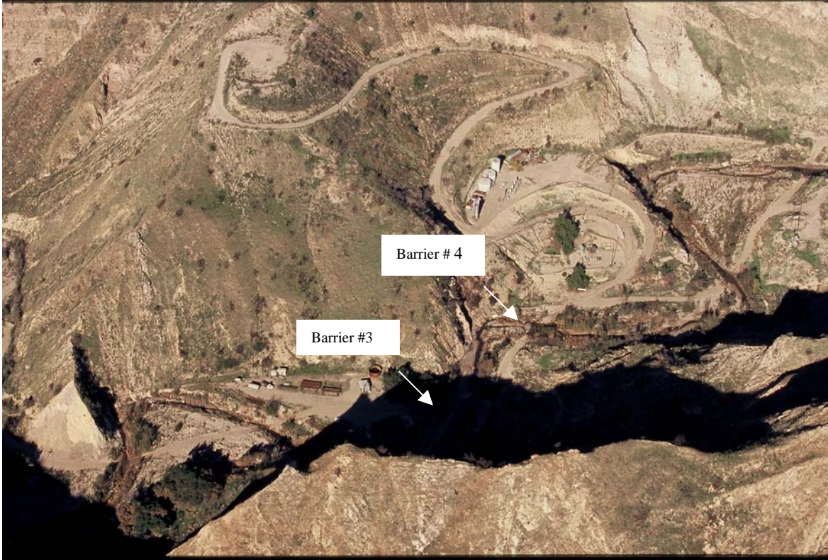
Hopper Creek Barriers #3 and #4 and other at-grade oil facility road crossings
