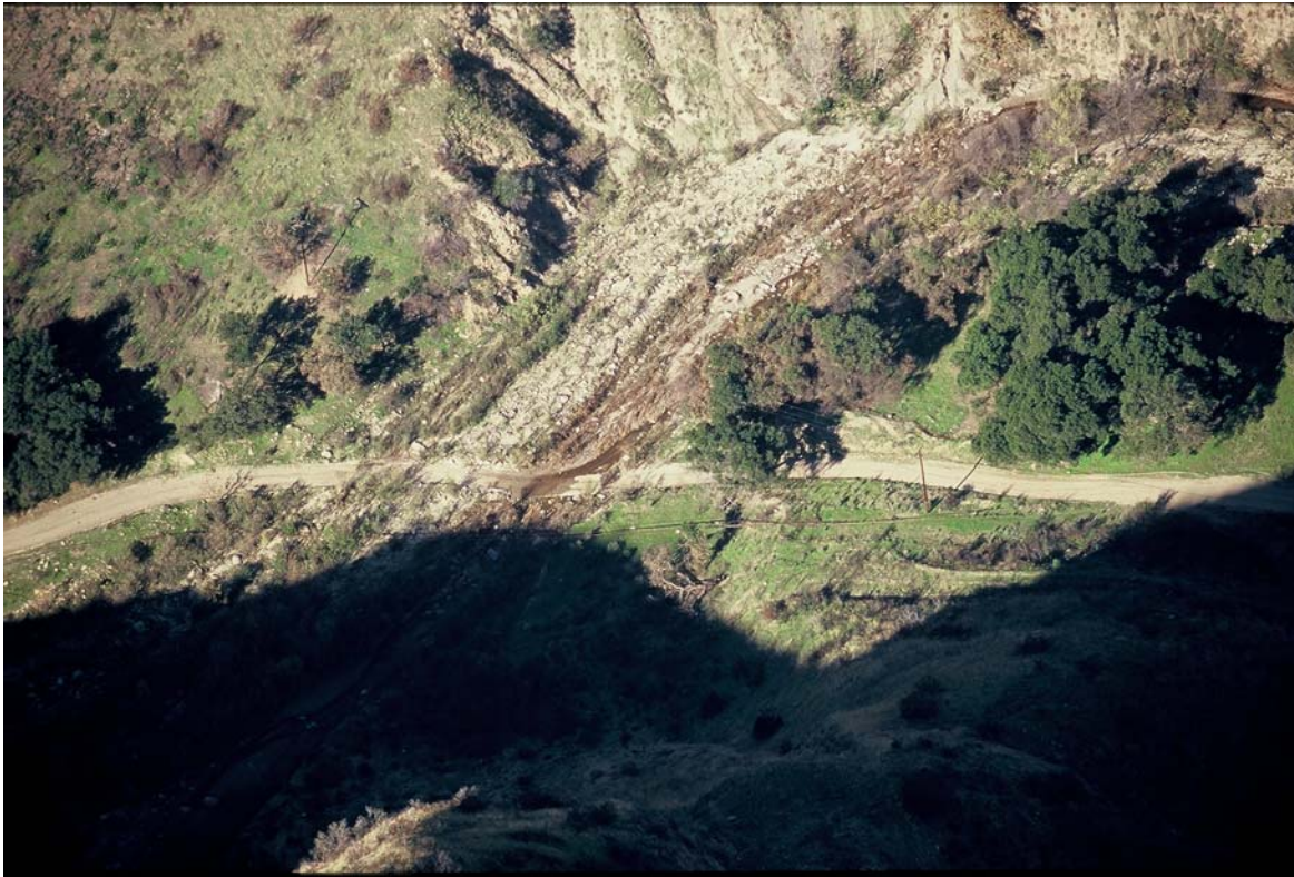
Hopper Creek barrier #2
