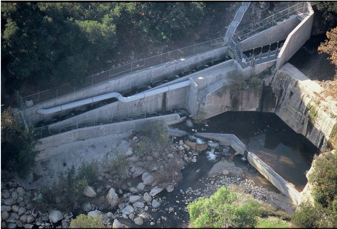
Dam and ladder before 2005 damage
