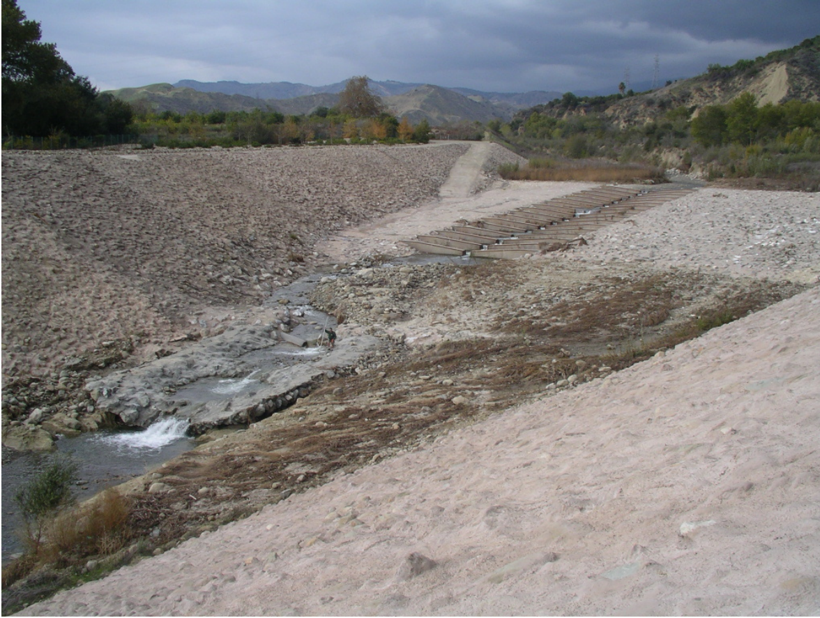
Grade control and fishway before 2005 failure
