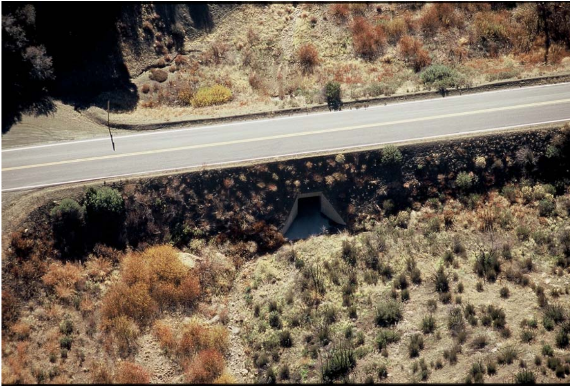
Burro Creek Highway 33 Box Culvert
